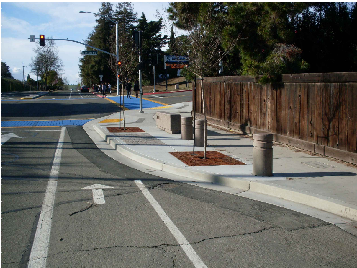
⑦ CORNER BULBOUTS THE SIDEWALK IS EXTENDED AT AN INTERSECTION CORNER. THIS IMPROVES THE VISIBILITY OF PEDESTRIANS AS THEY CROSS THE STREET, REDUCES CROSSWALK LENGTHS, AND ENCOURAGES SLOWER SPEEDS AS VEHICLES TURN RIGHT AROUND THE EXTENDED CORNER. THESE CREATE SAFER AND MORE COMFORTABLE CONDITIONS FOR ALL USERS AT INTERSECTIONS.
