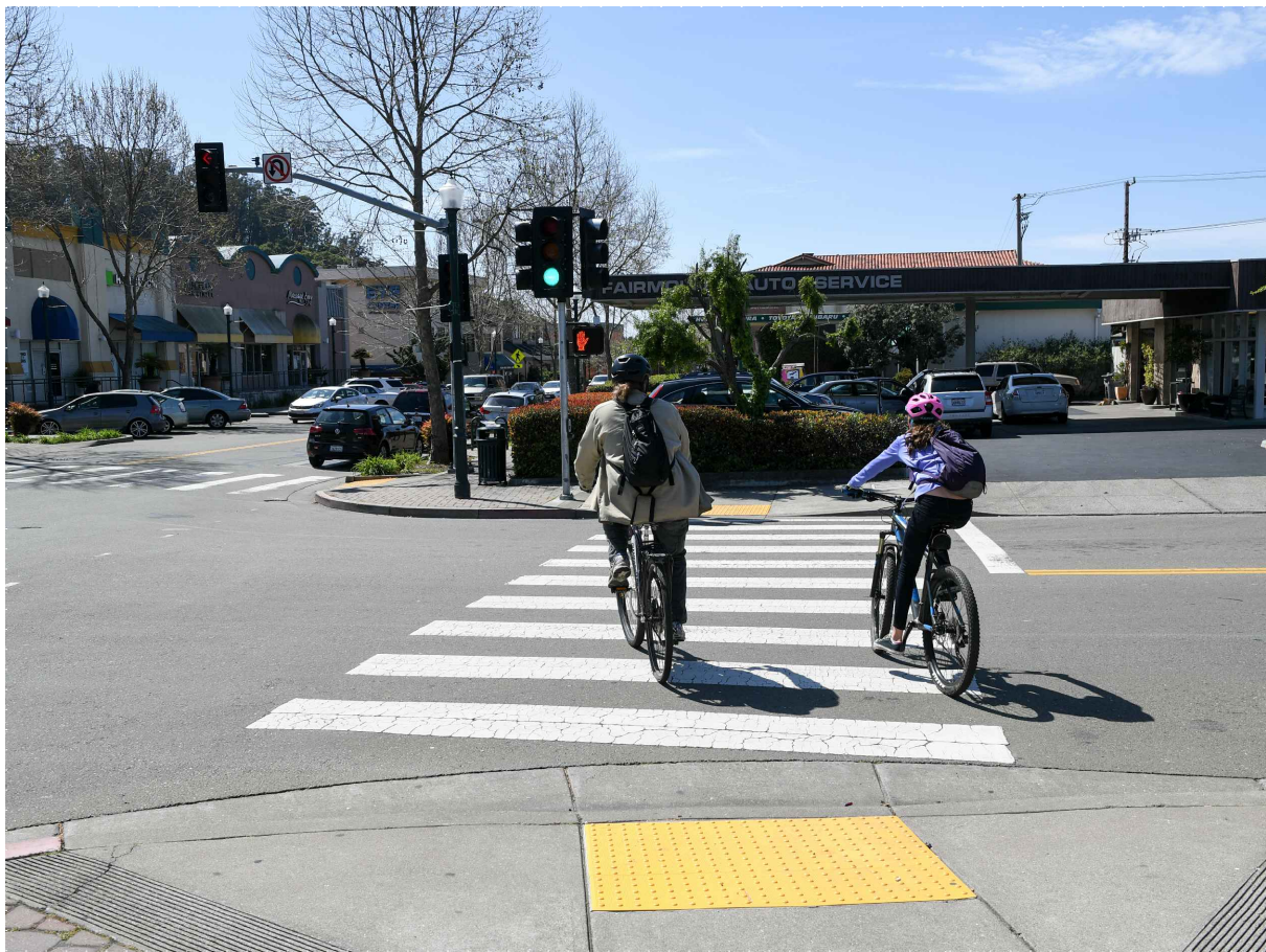
③ HIGH-VISIBILITY CROSSWALK PROMINENT AND VISIBLE CROSSWALK MARKINGS (USUALLY IN THE FORM OF A LADDER OR CROSSBARS AS SHOWN ABOVE) THAT HELP DRIVERS AND PEDESTRIANS BETTER IDENTIFY THE PRESENCE AND LIMITS OF A MARKED CROSSWALK. THIS ALLOWS DRIVERS TO BE MORE ATTENTIVE TO CROSSWALKS AND BE MORE LIKELY TO SEE PEDESTRIANS CROSSING.
