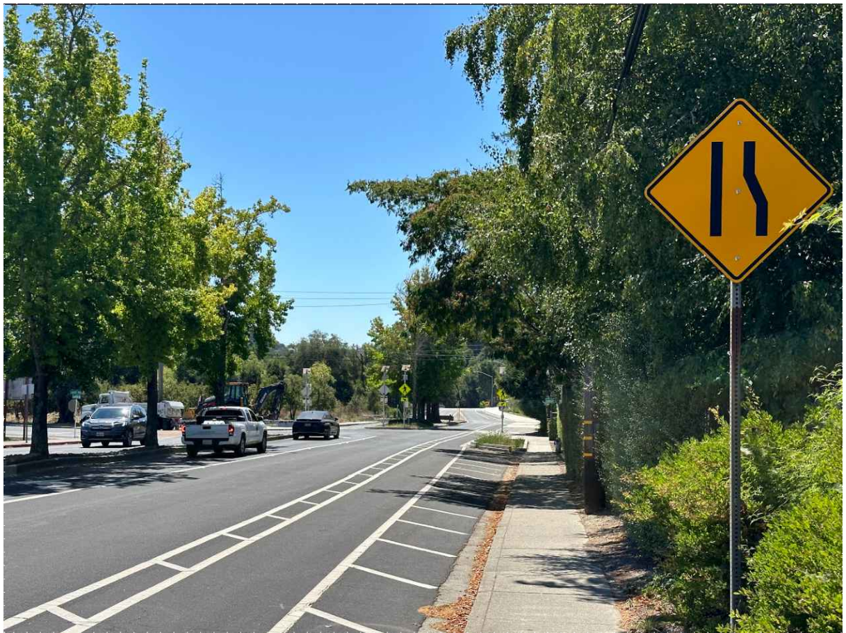
④ BUFFERED BIKE LANES TRADITIONAL BIKE LANES WITH THE ADDITION OF A STRIPED BUFFER THAT SEPARATES THE BIKE LANE FROM THE VEHICLE LANE. THIS SPACE SEPARATING THE LANES MAKES IT LESS LIKELY FOR VEHICLES OR BICYCLES TO IMPEDE ON THE OTHERS' LANE, MAKING A MORE COMFORTABLE AND SAFER FACILITY FOR BOTH USER TYPES.
