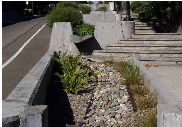
Stormwater management on a steep grade
