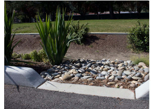
Erosion control next to parking lot on campus
