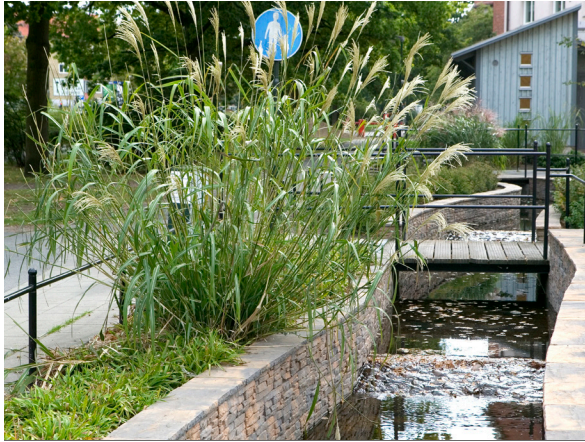
Stormwater management integrated into site design
