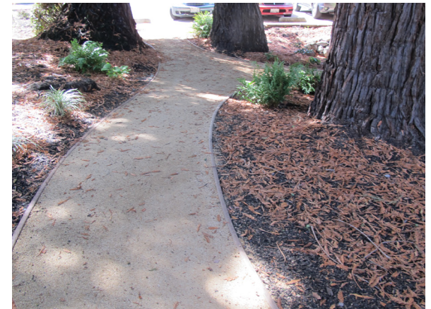
ADA compliant gravel walkway on campus
